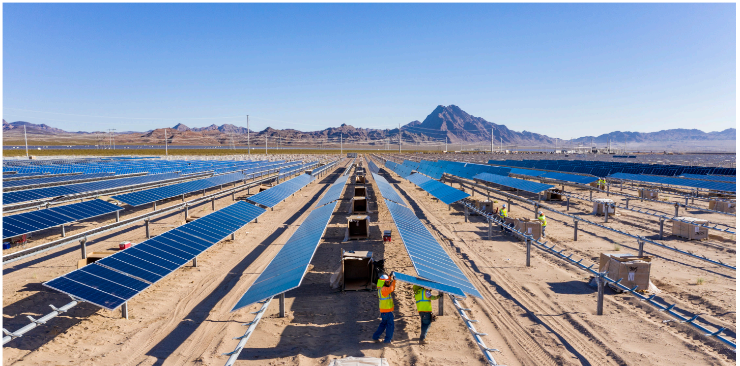
SRE at work constructing 251 MW in the Nevada desert.
